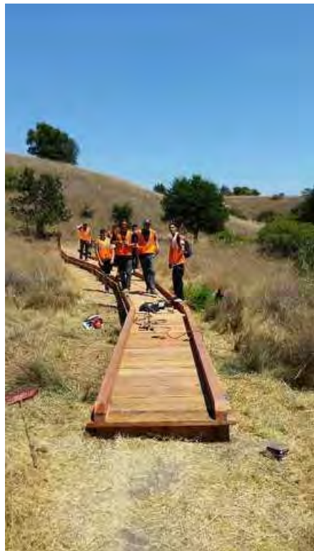
Youth Trail Crew repairing a puncheon crossing
