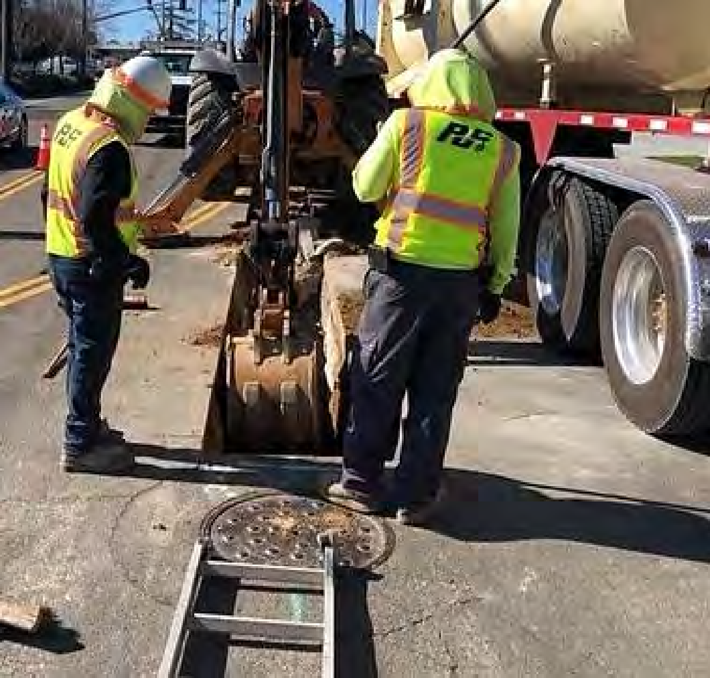
41 st Avenue at Soquel Drive Sewer Rehabilitation Project
