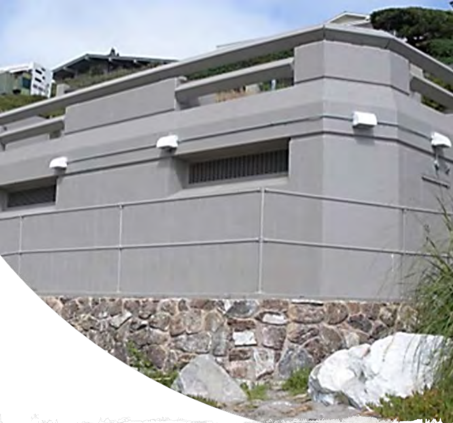
Hidden Beach Pump Station
