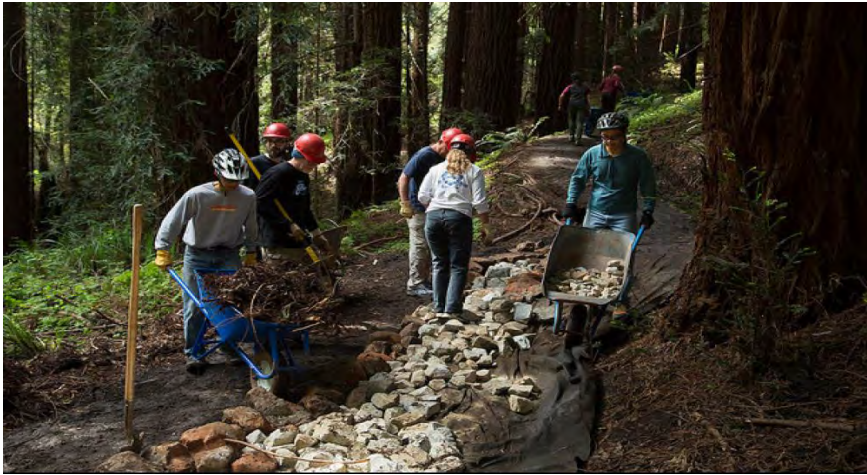
Volunteers repair erosion on the U-Con Trail, Pogonip Open Space
