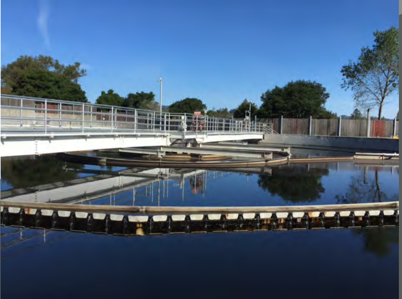
City of Santa Cruz Treatment Facility
