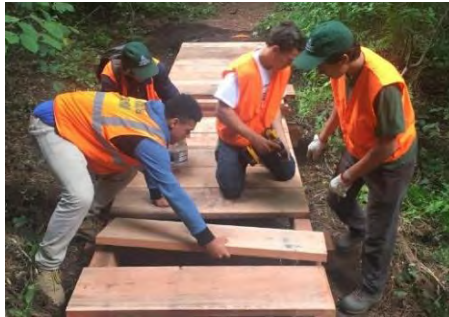
Bridge building and trail maintenance
