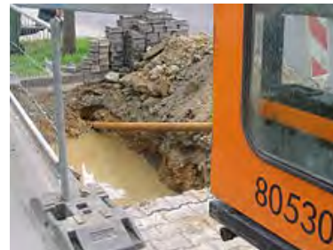
Starting pit with pilot hole and some drilling fluid in the pit.
