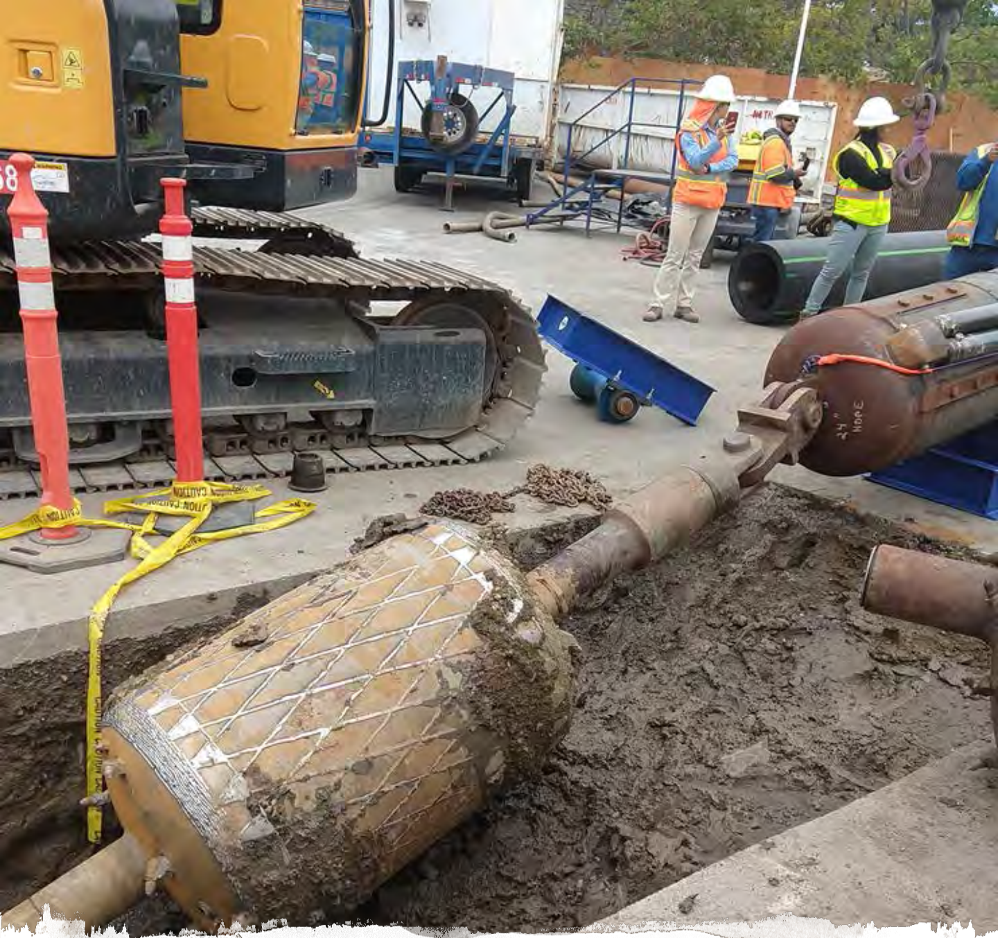
Soquel Pump Station Force Main Replacement Project Horizontal Directional Drilling
