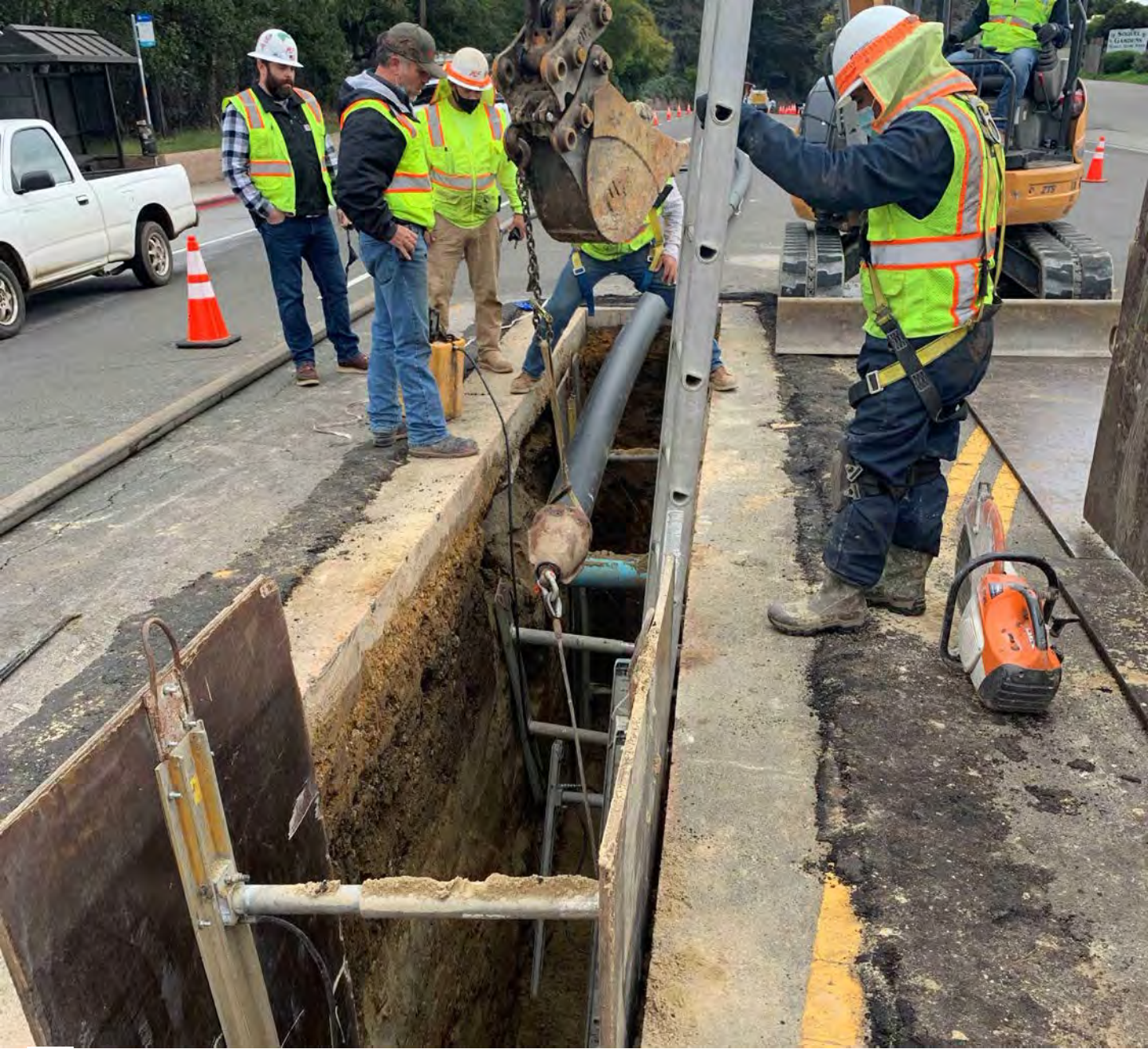
41 st Avenue at Soquel Drive Sewer Rehabilitation Project
