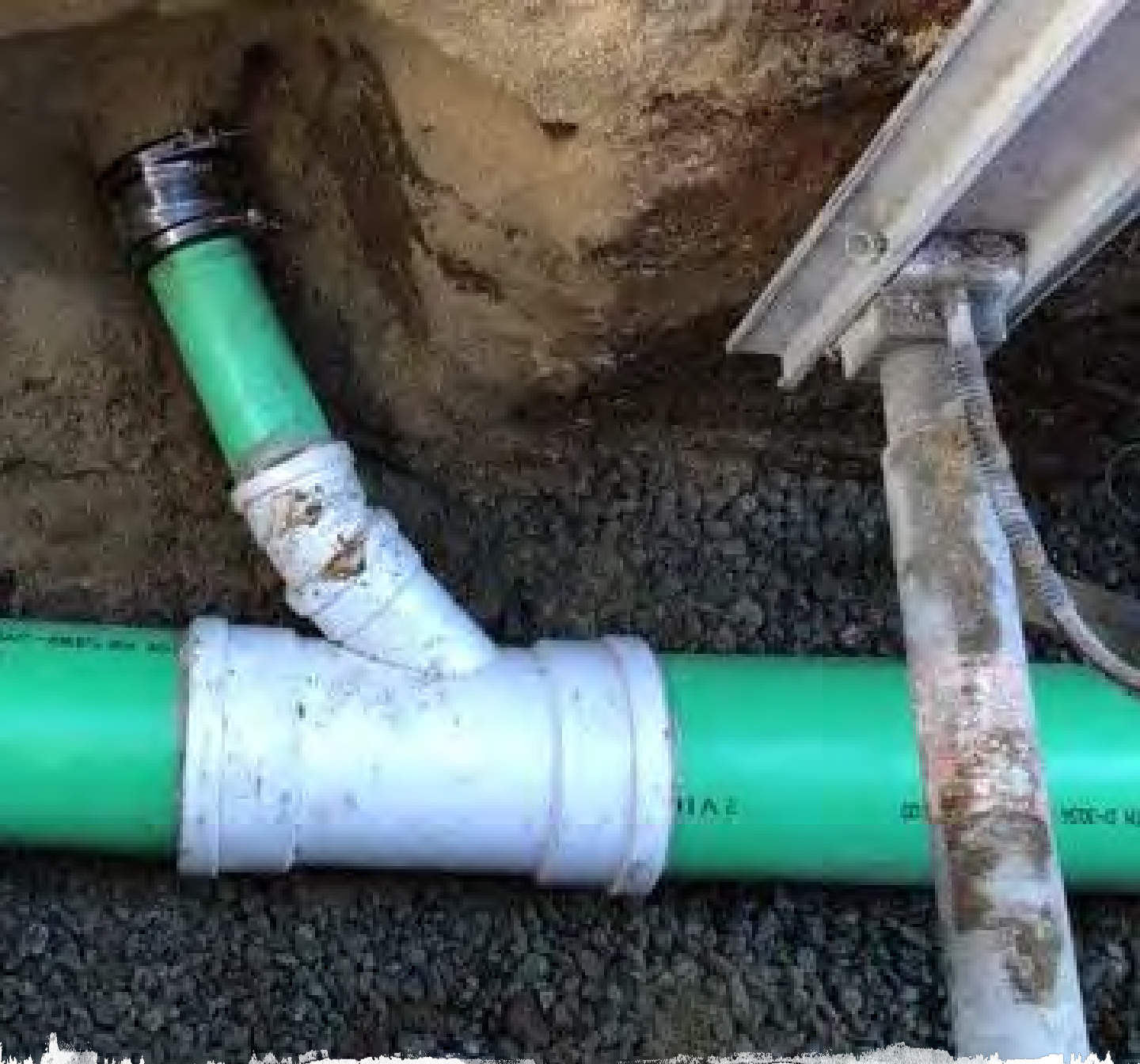
Cliff Drive Sewer Rehabilitation Project
